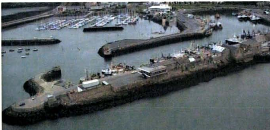
Figure 2: Western elevation of pier (MWP)
