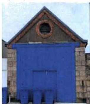
Figure 17: Former Lifeboat House
