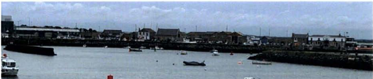
Figure 21: Howth Harbour - View towards West Pier from East Pier
