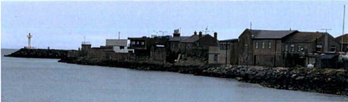
Figure 24: Rear elevations of buildings on West Pier, viewed from south west
