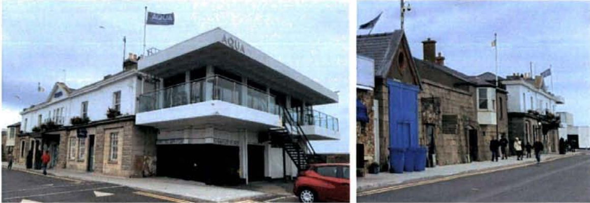
Figure 19: Former Harbour Master's House
