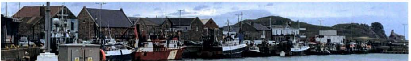
Figure 15: Protected Structures on West Pier, viewed from south of harbour
